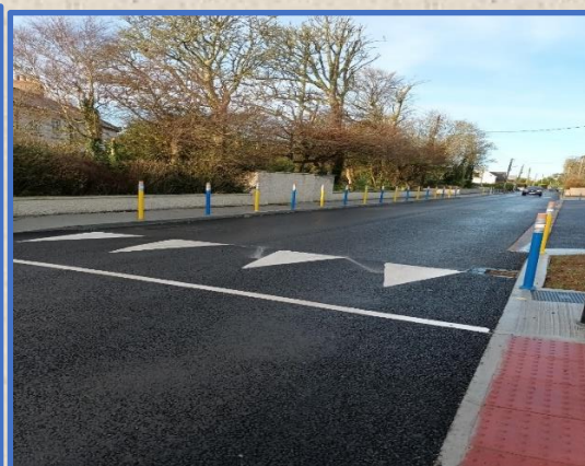
Works at St Mary's National School, Rosslare Strand
