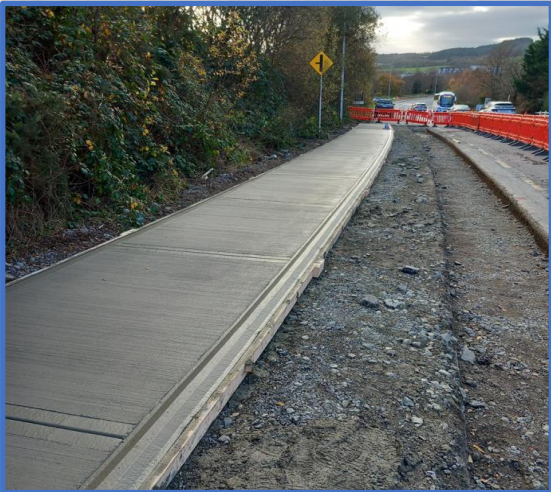
Construction of the segregated cycle and pedestrian scheme at Newtown Rd
